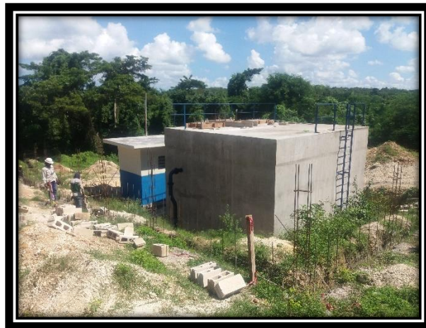
Nonpariel W.S.S., Westmoreland - Construction of Pumping Station
