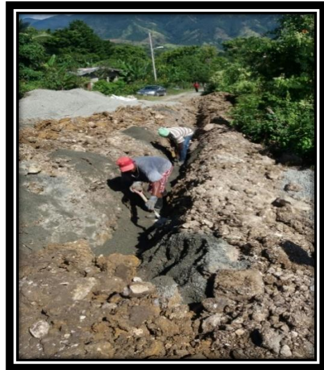
Georgia WSS – Men preparing trench for the installation of pipeline
