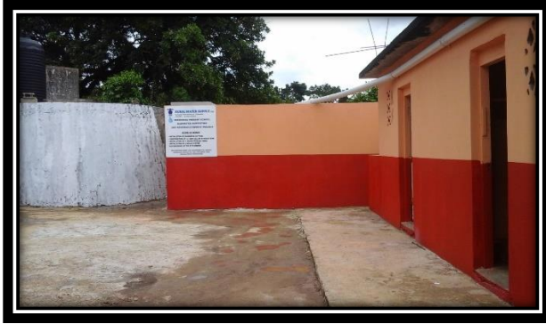
Beersheba Primary School, St. Elizabeth - 16,000 gallon Ferro-cement Tank completed
