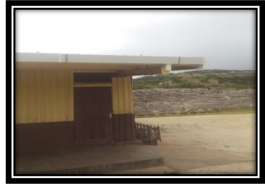
St. Mary's Primary School - New Gutter Installed
