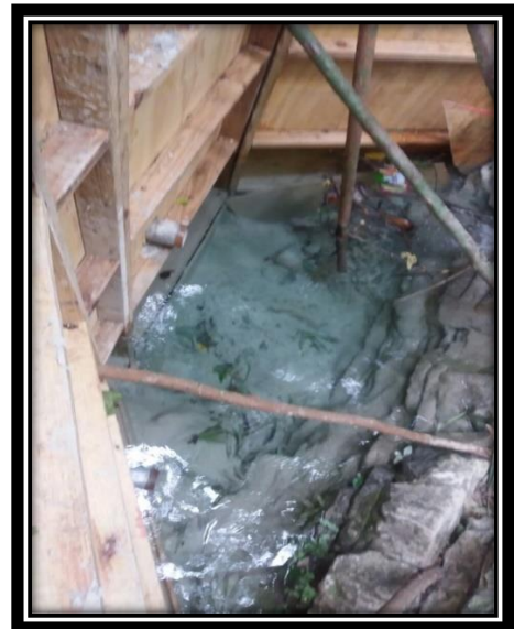
Georgia WSS – Dam Construction
