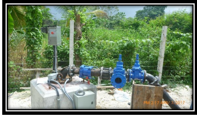
Montpelier Well Rehabilitation, St. James - Installation of Submersible Pump
