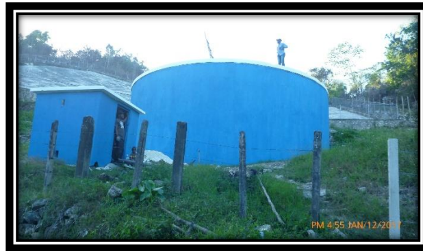
Thompson Hill Catchment Tank (after rehabilitation)
