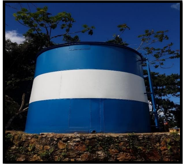
McNie Water Supply System, St. Ann - 50,000 Gallon Steel Tank
