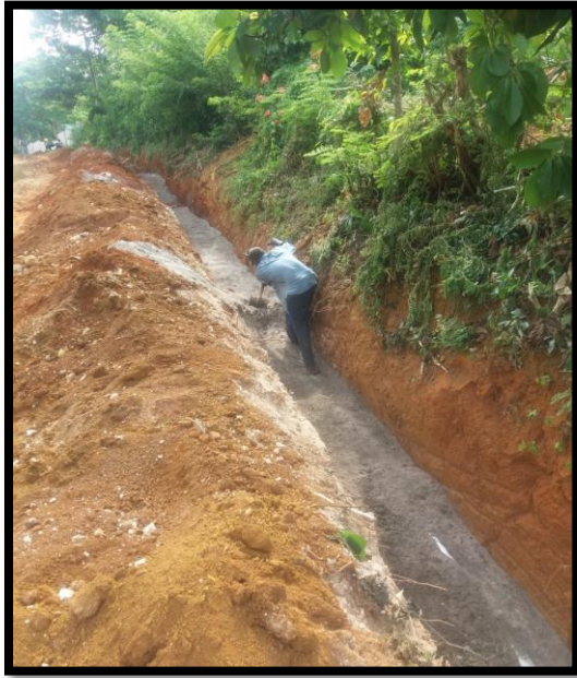
Top Reading Water Supply System, St. Elizabeth - Bedding of pipeline
