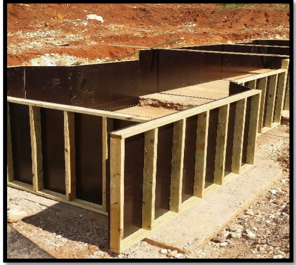
Kennedy Grove Water Supply Treatment Plant, Clarendon - Construction of Grit Channel
