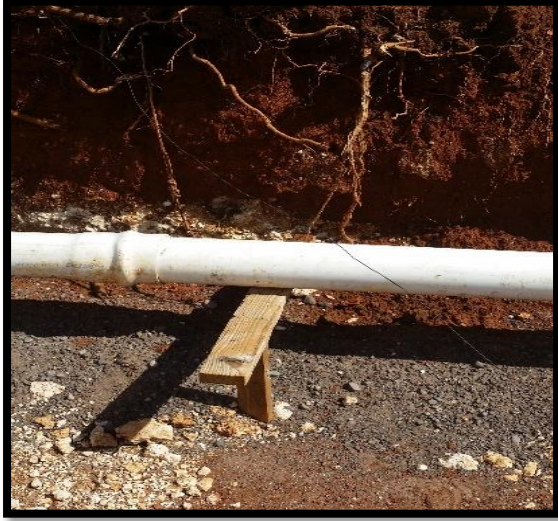
Kennedy Grove Water Supply Treatment Plant, Clarendon - Construction of Force Main
