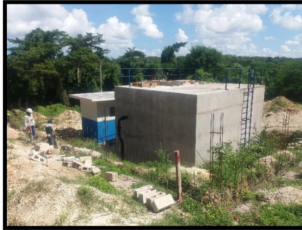
Nonpariel Water Supply System, Westmoreland - Construction of Pumping Station
