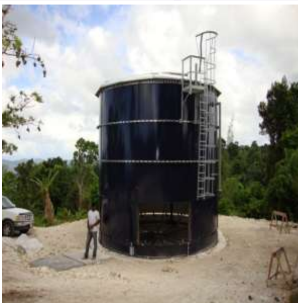
Hunts Town Water Supply - Storage Tank under construction
