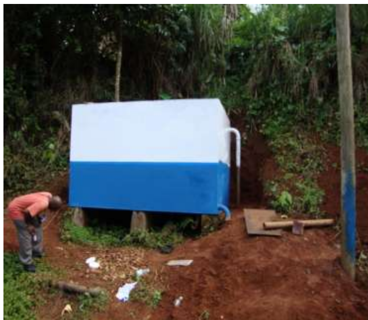
Waugh Hill Relift Pump Feeder Tank - After
