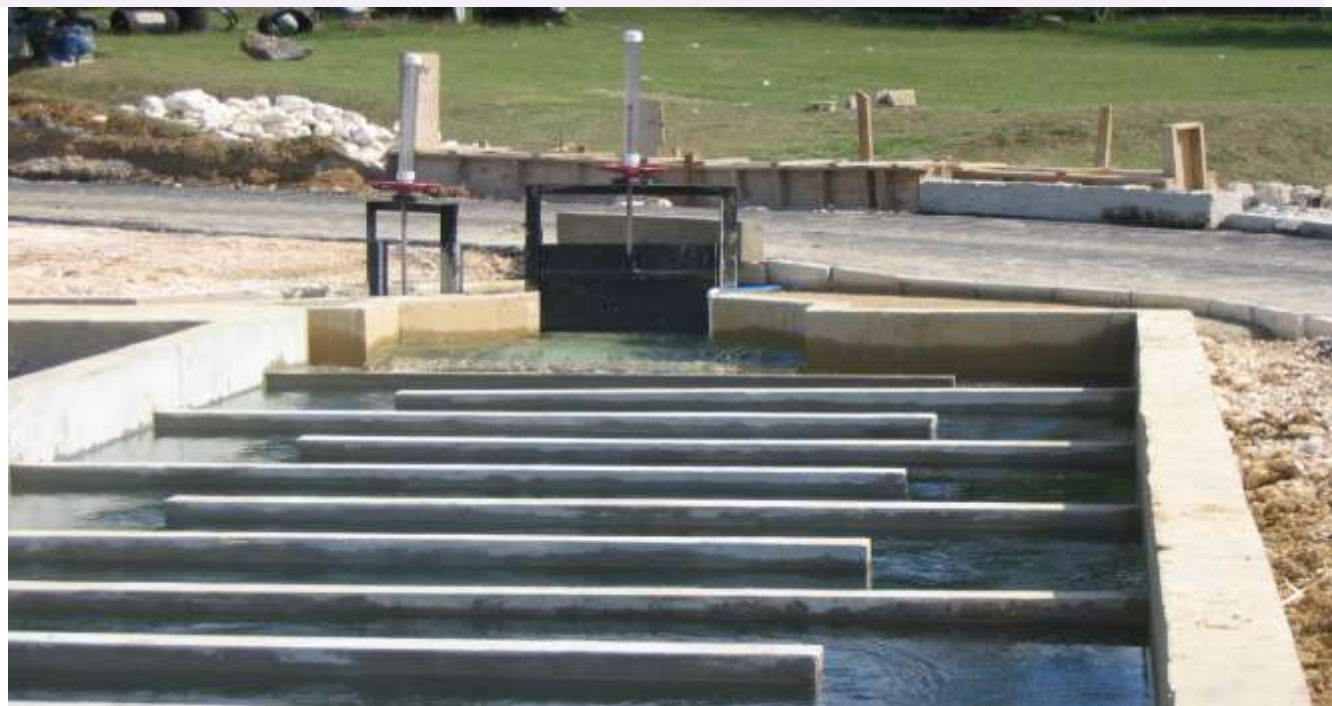
Roaring River – Clari-Flocculator.
