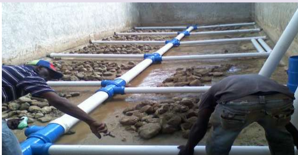
Peace River Filter Repairs
