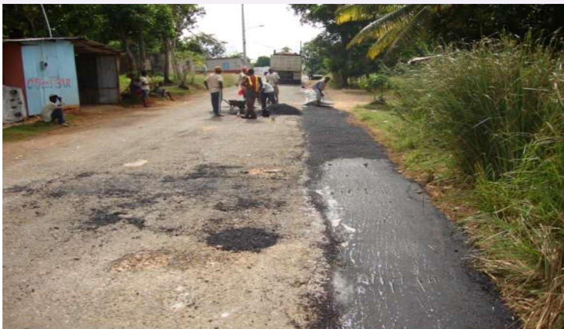
Macca Tree Water Supply - Road Reinstatement
