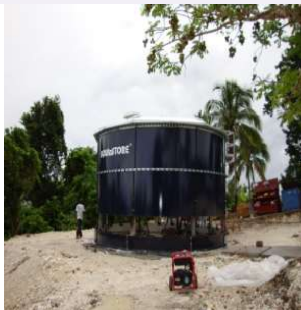
Hunts Town Water Supply - Storage Tank under construction
