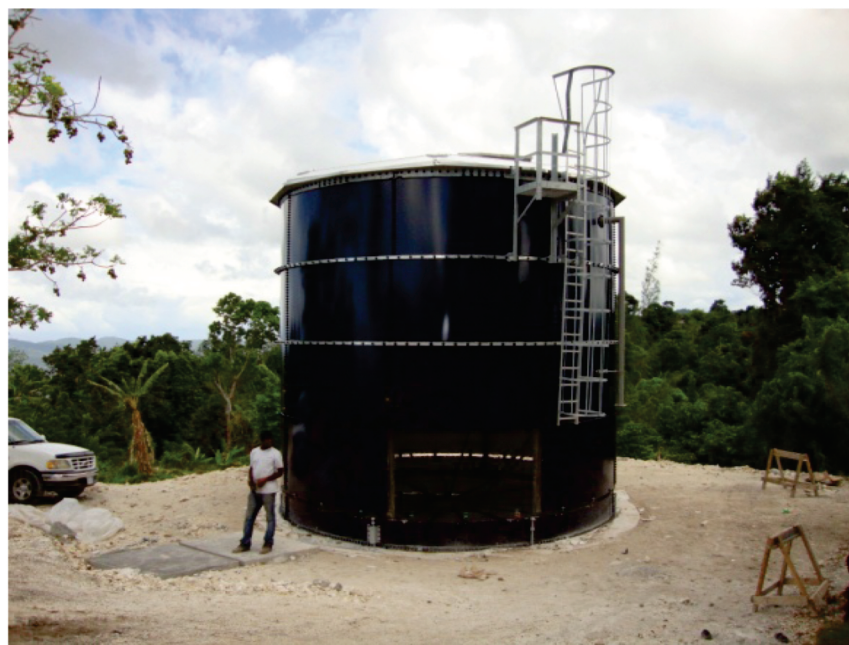
Hunts Town Water Supply - Storage Tank under construction
