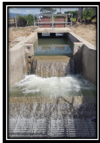
Artificial Recharge Project – Inlet Chamber and Bar Screen
