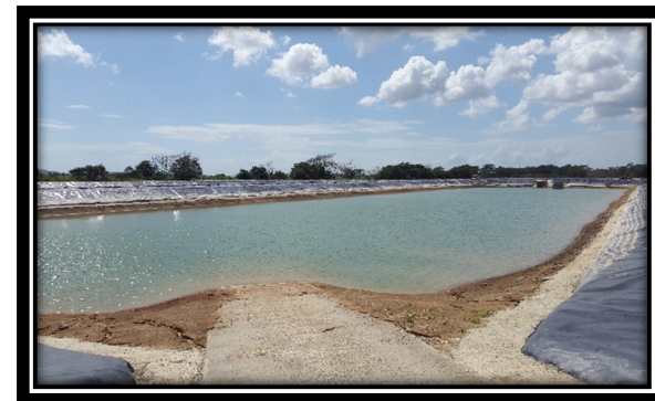
Artificial Recharge Project – Settling Basin
