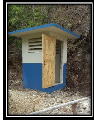
Llandewey Water Supply, St. Thomas – Chlorine House
