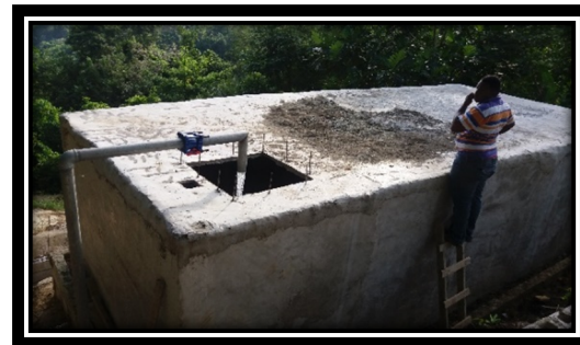
Pear Tree River WSS, St. Thomas – Ferro Cement Tank (After)
