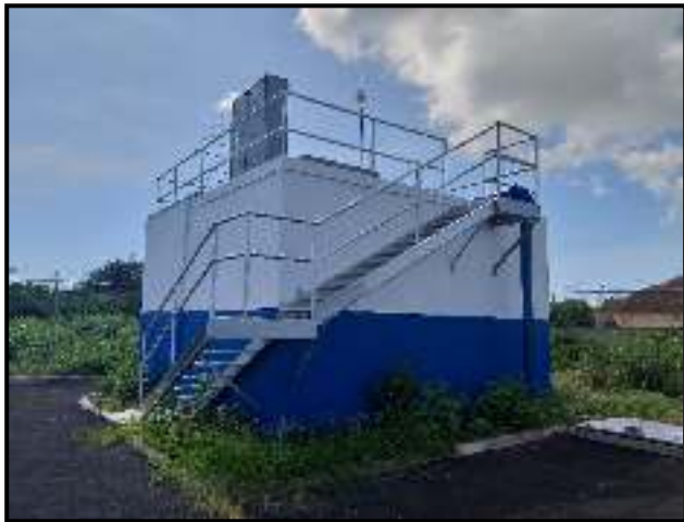
Portland Cottage Pumping Station, Clarendon
