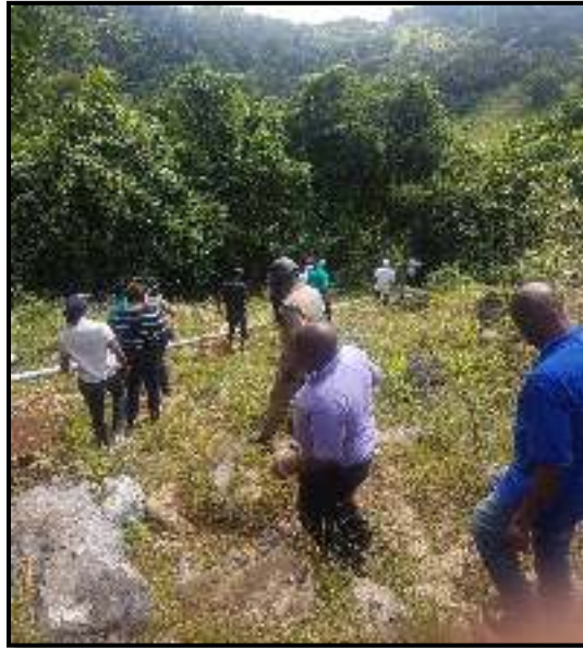
Spring Gardens Pipeline
