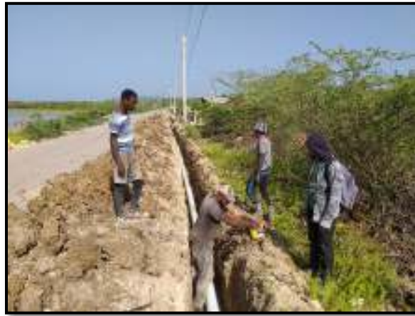
Pipelaying activities at Portland Cottage, Clarendon
