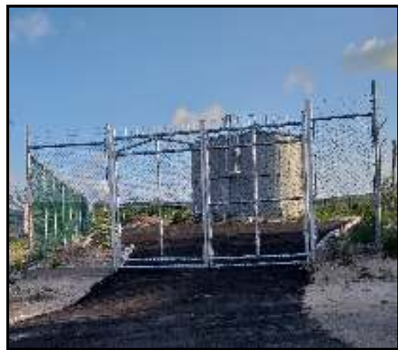
64,000 gal. Reservoir at Portland Cottage, Clarendon
